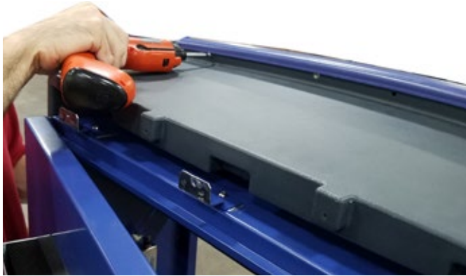
Figure 16. Attach Blue Roto Mold #4 with (3) screws to gray Roto Mold #3
