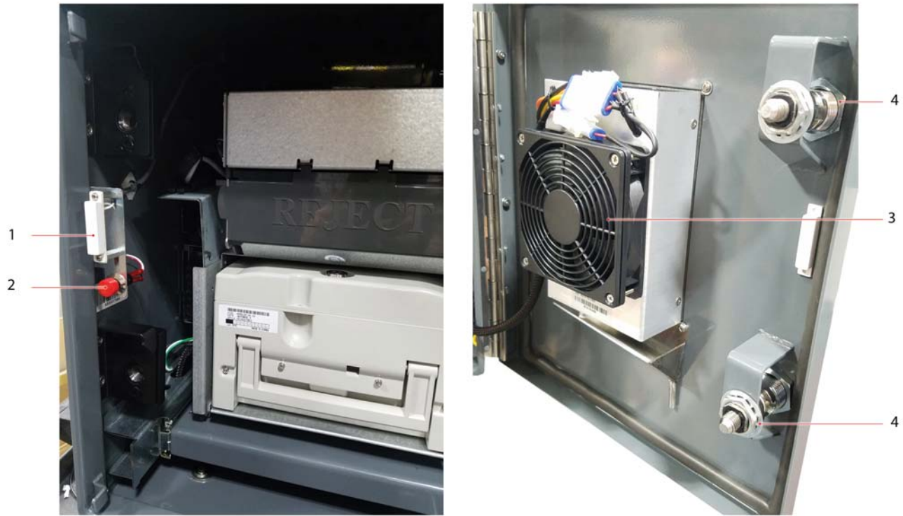
Figure 22. CPT Interior Base
