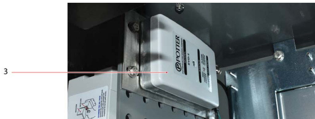
Figure 18. Upper-right Chamber with Vibration Detector
