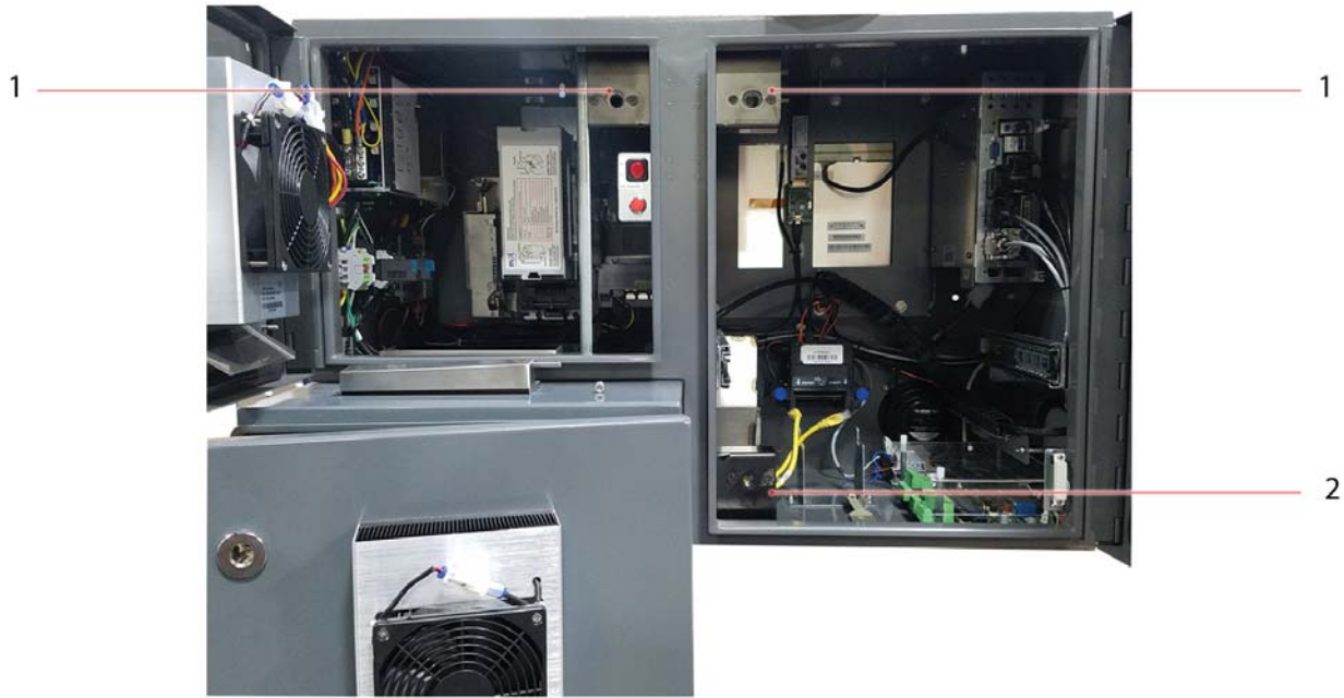
Figure 20. Security Locks in Upper Chambers
